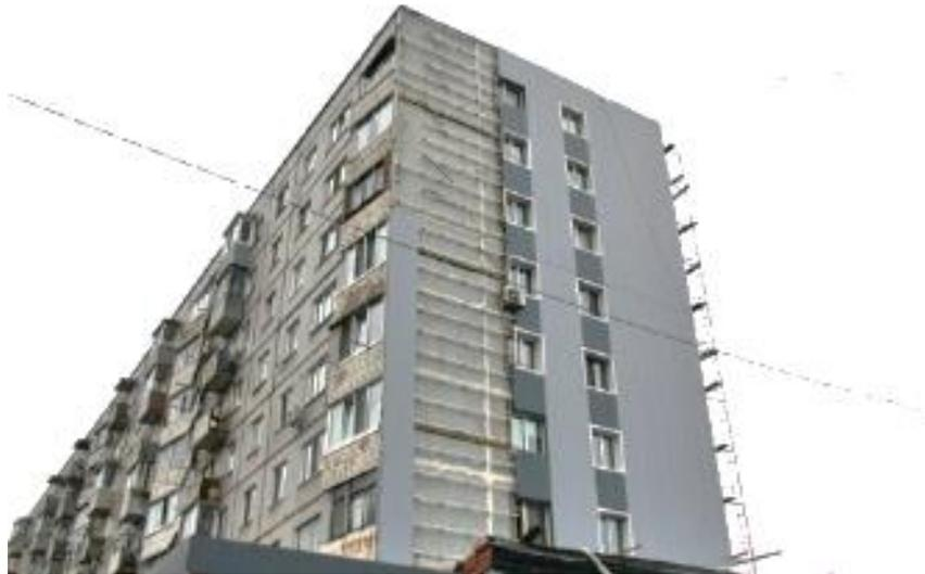
Figure 4. Insulating the envelope of a large-panel building using a ventilated façade
