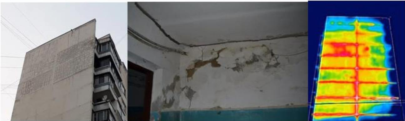
Figure 1. Defects of panel houses
