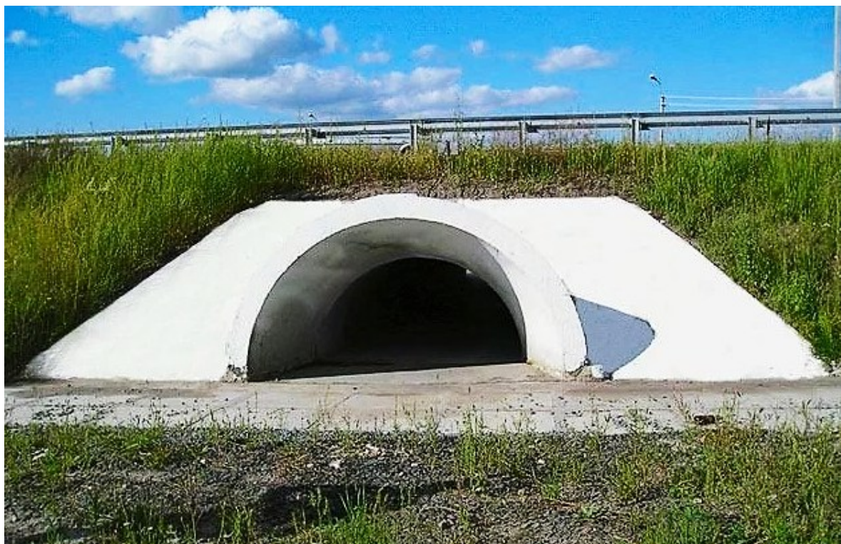
Figure 1. Culvert structure of the highway
