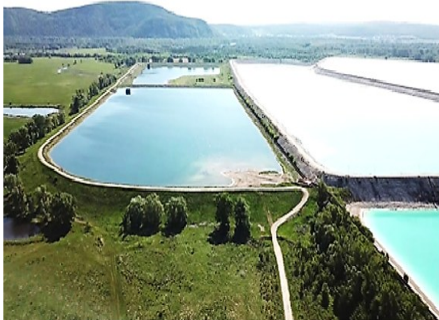
Figure 2. Sludge accumulators of the “Bashkir Soda Company” (aerial photography, Sterlitamak)
